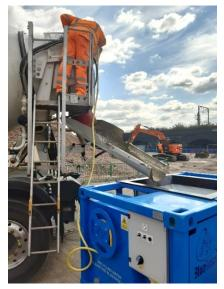
The solids will be caught in the Nappy Sack, the pH of the water will be reduced as it passes through the sack and drains into the sump where it returns to the tank, forming a closed loop.
